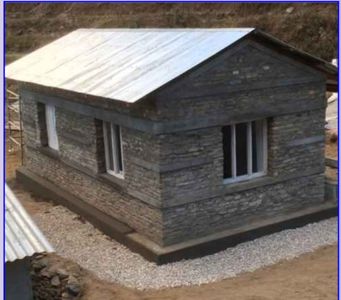
A new house for a Welfare pensioner in Pachok
