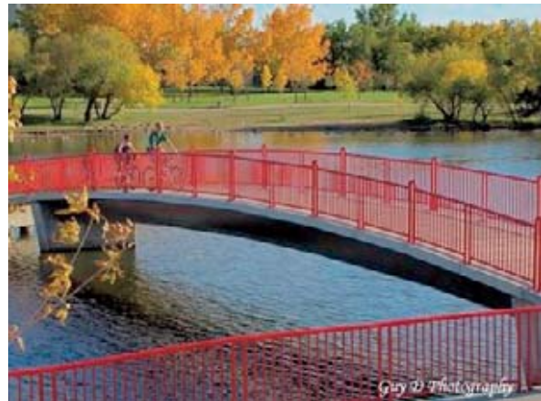
Wascana Centre Authority constructed the Broad Street Bridge in 2009-2010 for cyclists and pedestrians to avoid a busy road bridge. Photo courtesy of Guy D. Photography, Regina.
