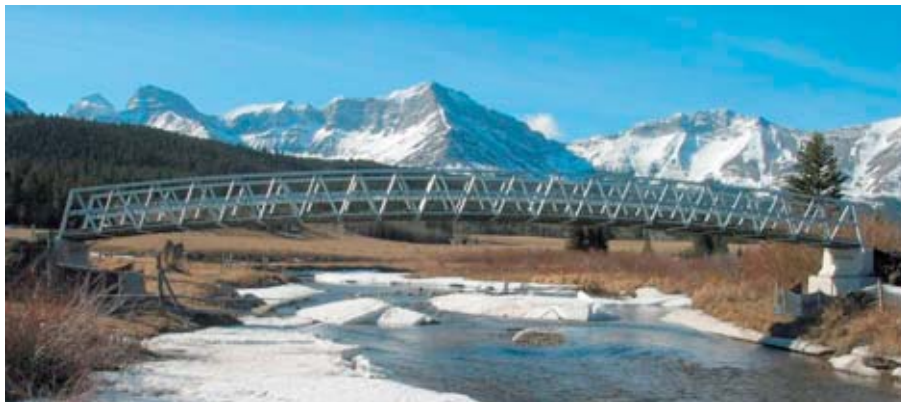
Shared use trail bridge over the Crowsnest River in Southern Alberta.
