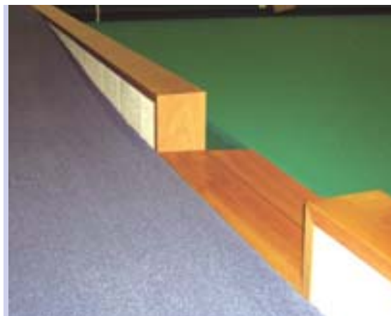
Ramped side surround
