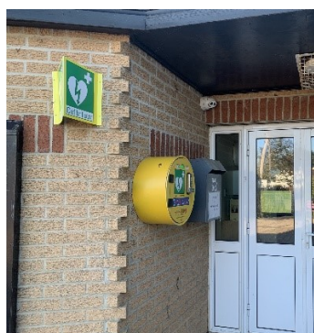
Needingworth Village Hall
