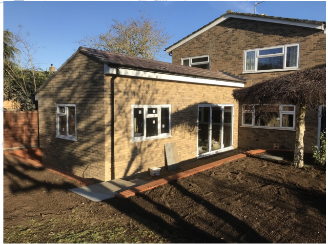
Extension in progress, 2023
