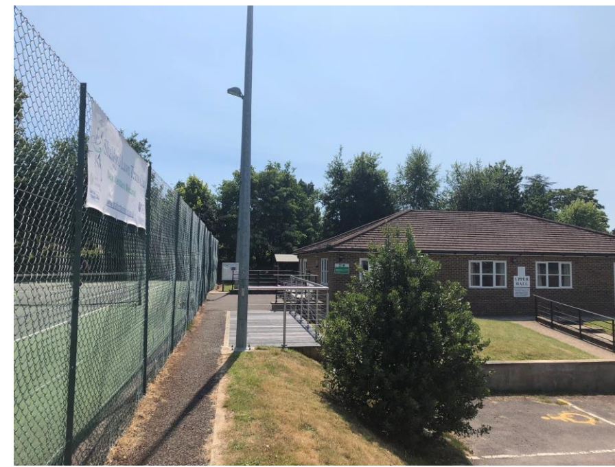
Figure 12: View towards the development site taken from top of steps at NW corner of tennis courts
