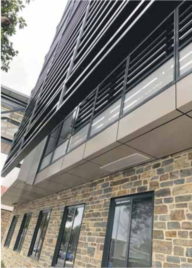
EYES ON THE PAST... Stone from former main campus buildings has been used in the frontage of the building.
