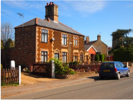
Many buildings in Denver are built from the local carrstone. Image by Sheils Flynn for OWLP.
