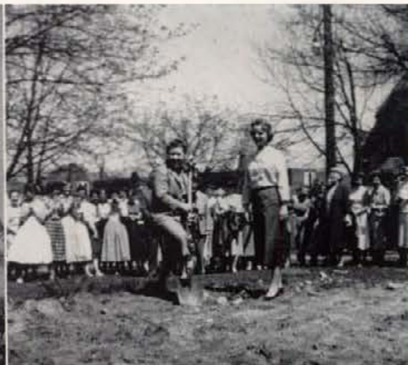
Ground Breaking Ceremony
