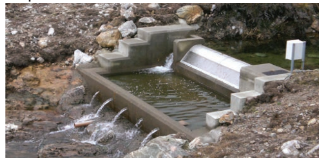
micro-hydro power generation
