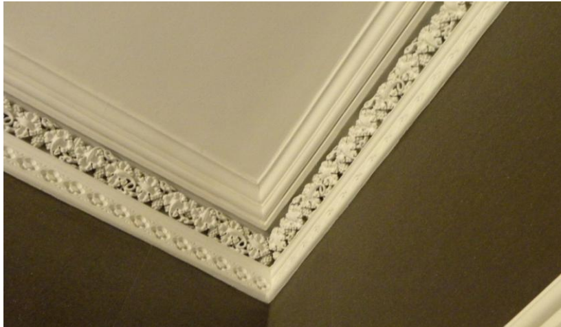
Detail of the cornice
