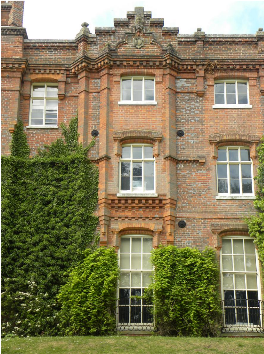
The eastern elevation of Hughenden Manor showing window treatments with basket arches, brick corbelling and dentils and a heavy ornamental parapet hiding the roofs.
