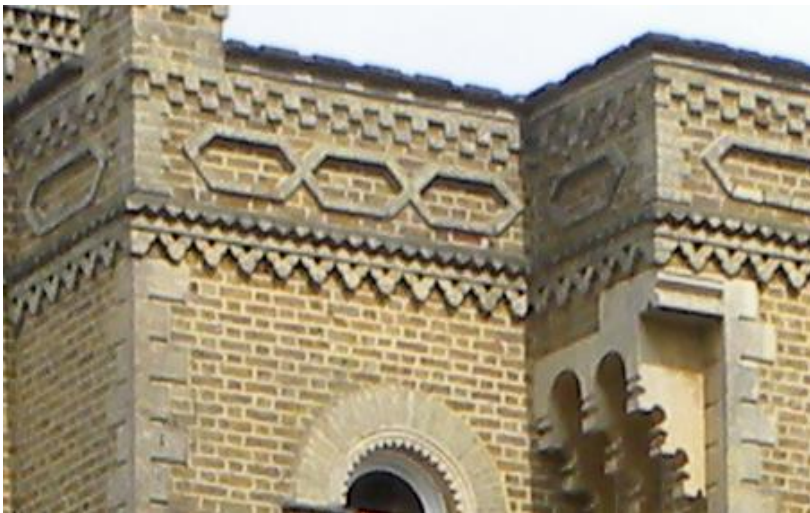
The tower parapet
