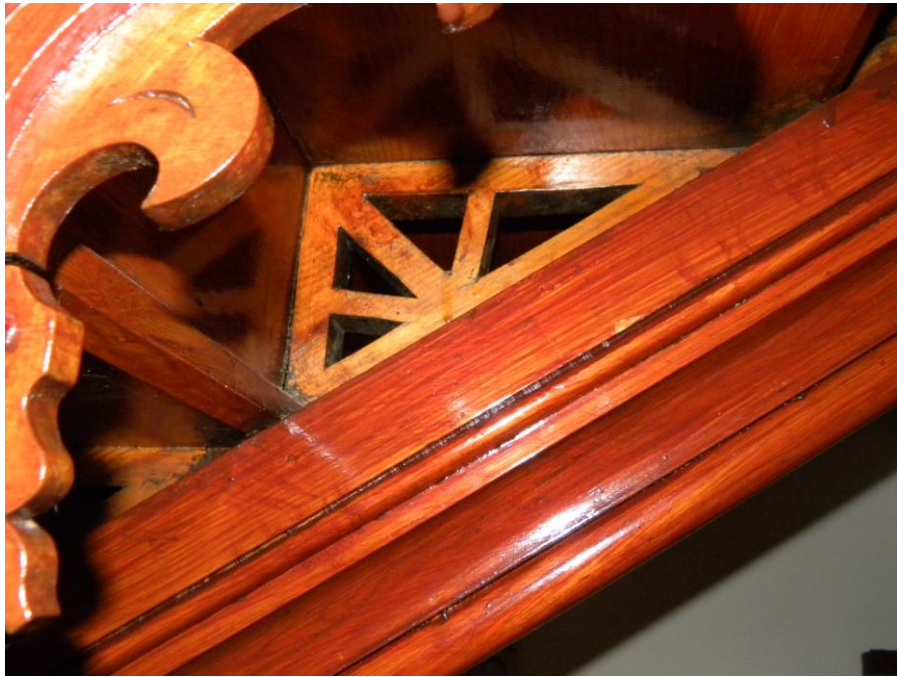
Detail of the brackets under the stairs
