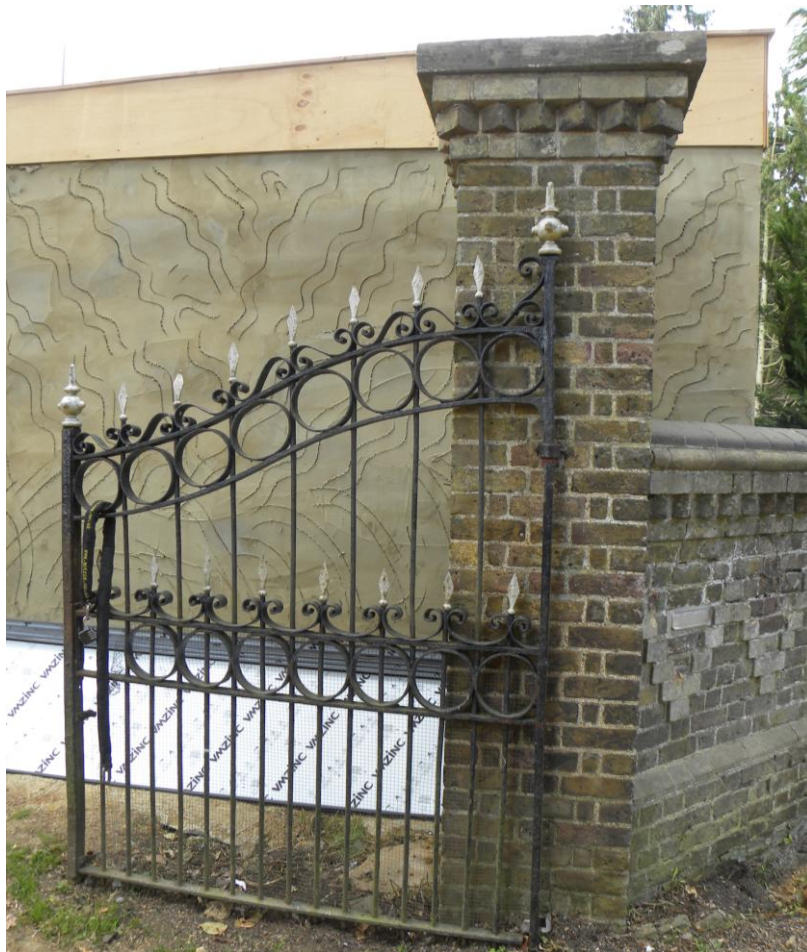
Historic boundary walls,, gates and gate piers of the former St. Huberts Lodge (May 2011)
