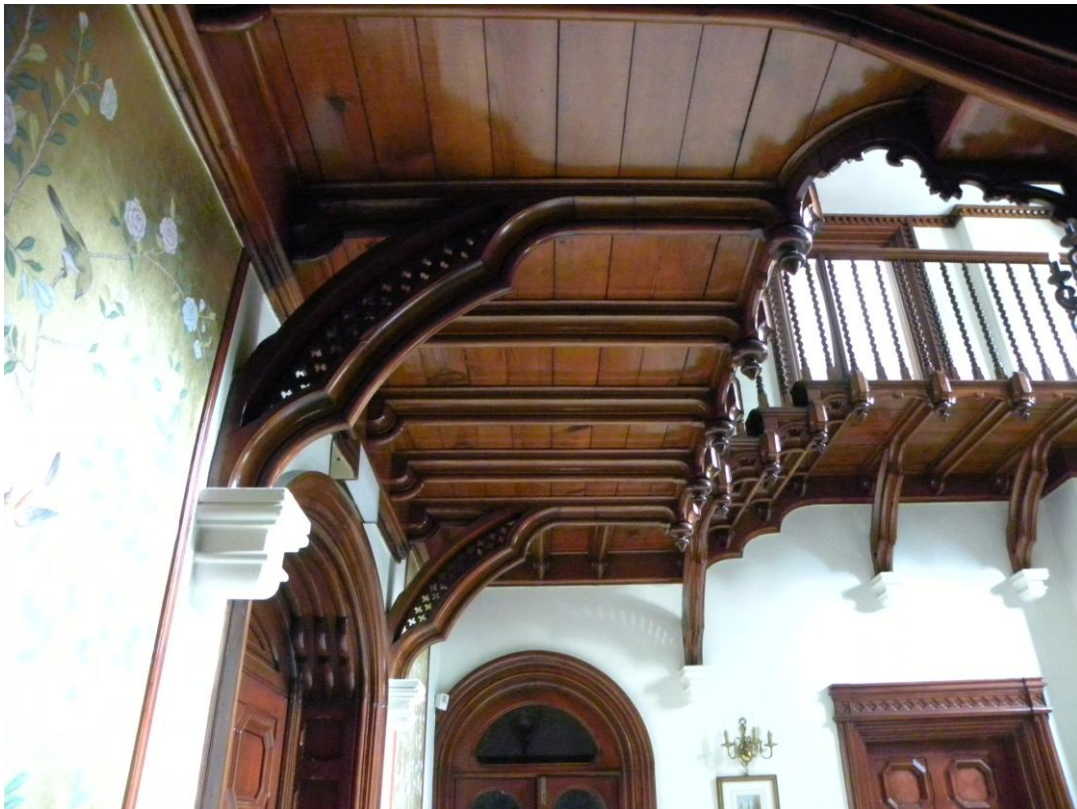
Detail of carved brackets, twisted balusters and carved pendants underneath the landing.
