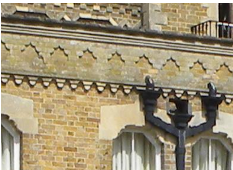
The four-bay extension parapet
