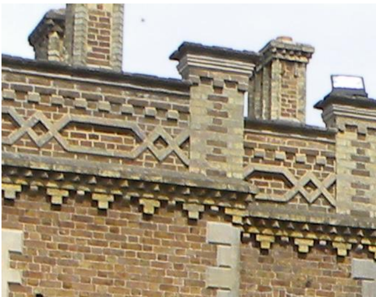
The west wing parapet
