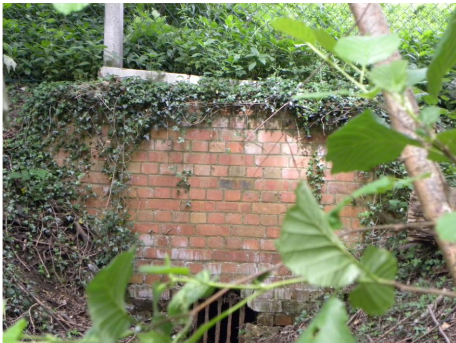
The red brick English bond retaining wall – the stream runs through the grid beneath. Photograph taken looking north towards the A40.
