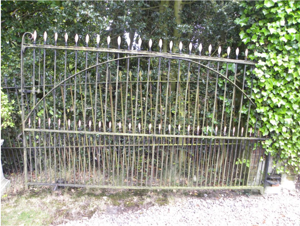
The “Baldwin” gate with park railings behind.
