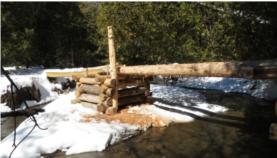
New footbridge under construction at km 8 of GHTA trail.
