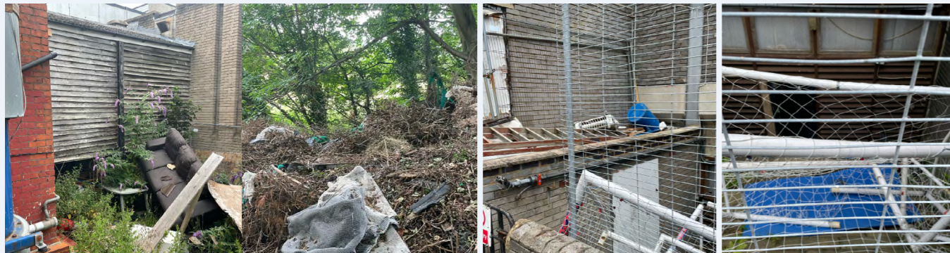
WASTE TIPPED BEHIND KITCHEN & BY TENNIS COURTS
