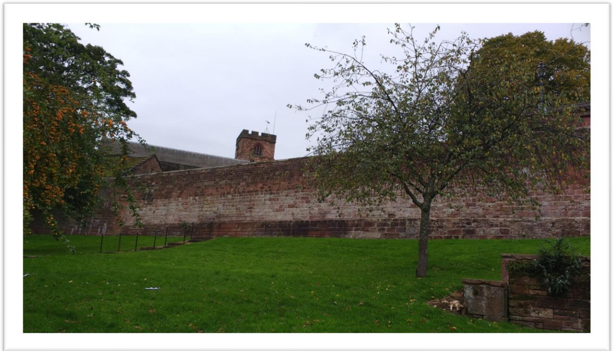
Figure 6. Looking up to the Cathedral Close from Town Dyke and the Caldew. The wall is about four to five metres high from this side, but only about a metre high on the Cathedral side. The Blackfriars Street strip houses ran back to this edge just to the right of the picture.
