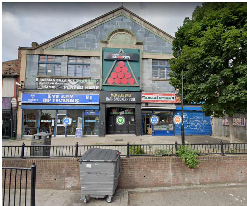
Figure 2: Existing site frontage
