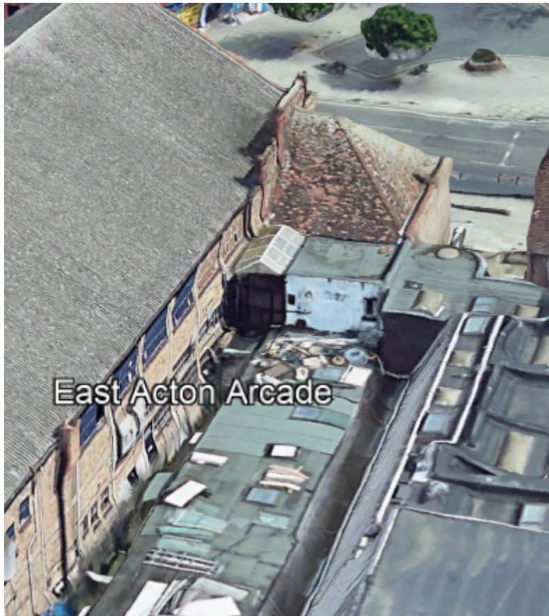
Figure 12: Rear elevation of 91 Old Oak Common Lane
