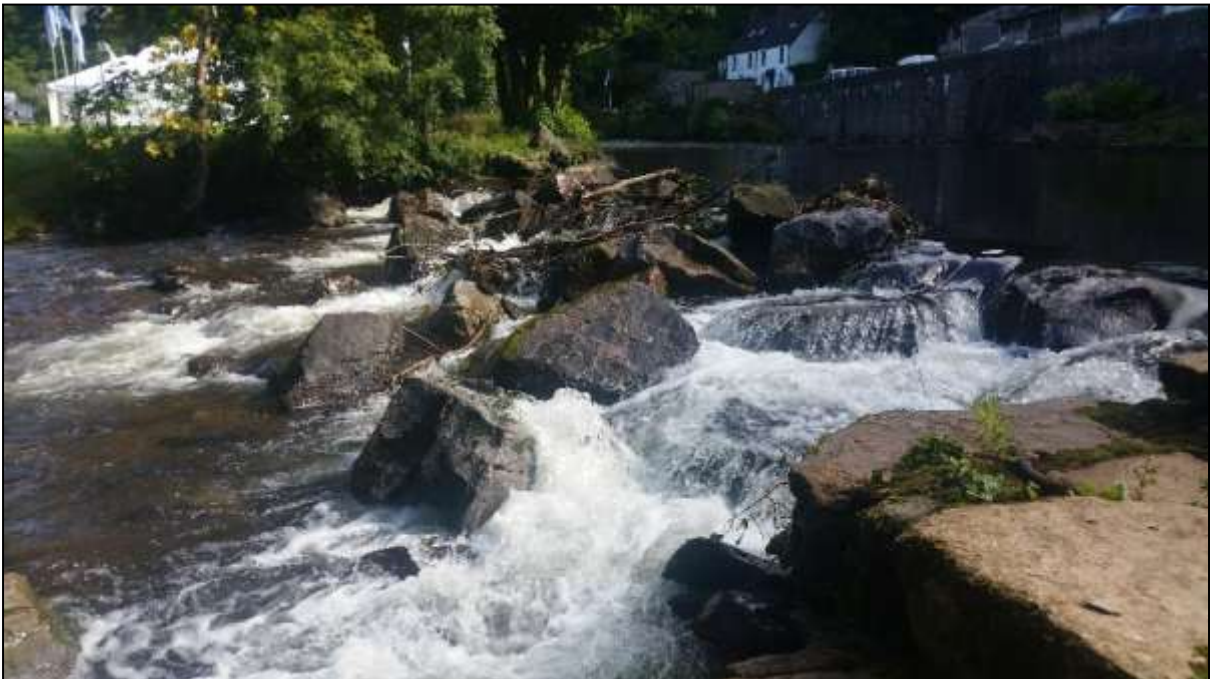
Figure 16: The nature-like fish pass on Dulverton Weir.
