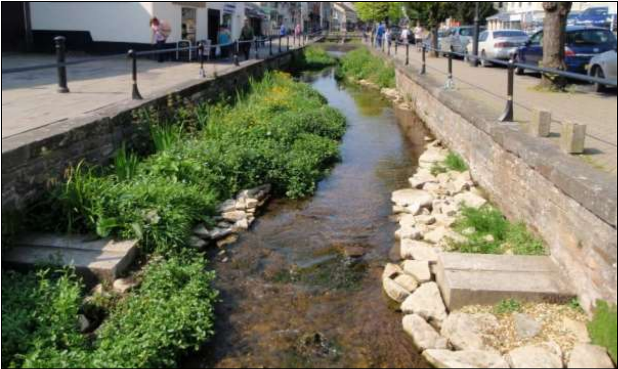
Figure 26: Planted stone berms in a hard-engineered channel in Midsomer Norton, Somerset
