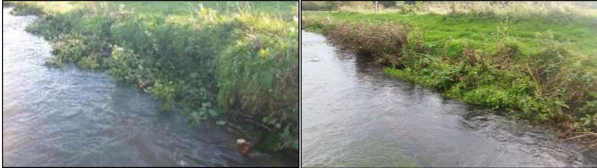
Figure 24: A marginal brushwood shelf immediately after installation (left) and after one year (right)
