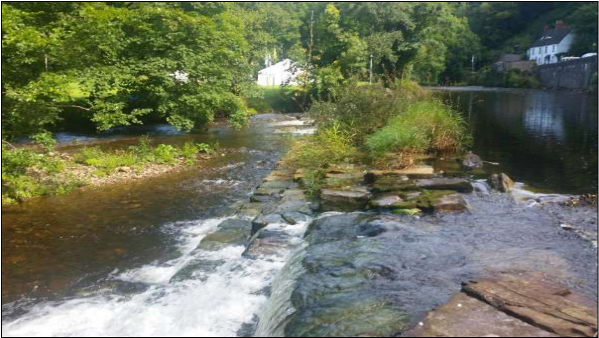
Figure 17: The blockstone (middle) section of the weir
