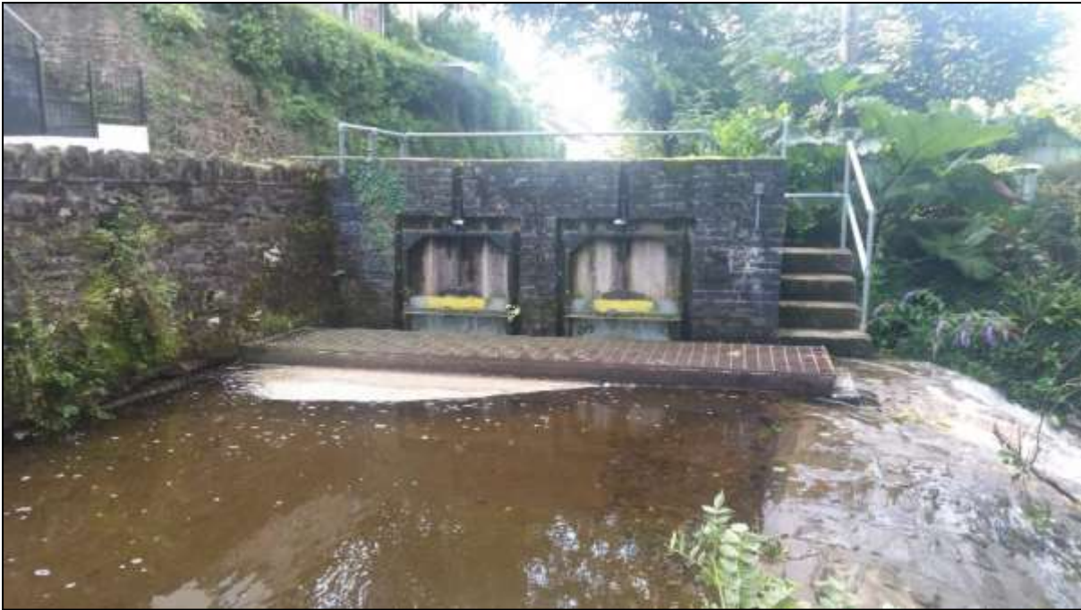
Figure 15: An view from upstream of the undershot sluices
