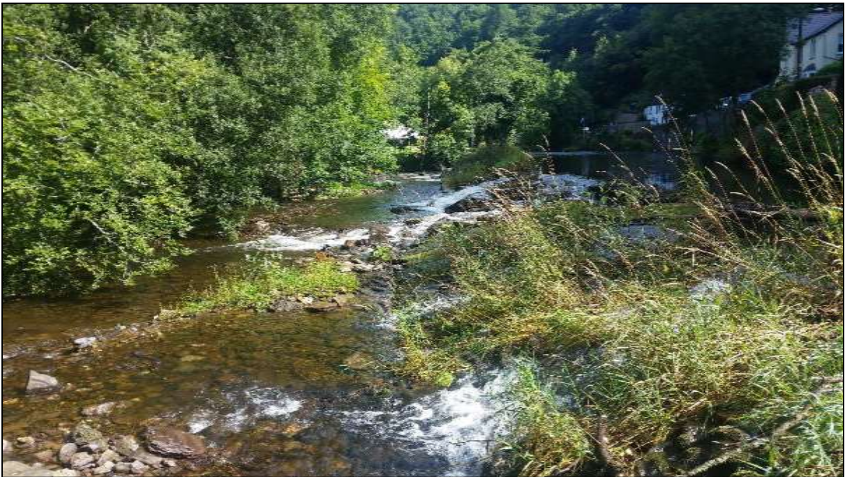
Figure 18: The oldest part of the weir constructed from wooden stakes and hand-placed stones.
