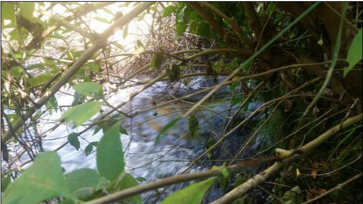
Figure 3: The culvert discharges over a shallow concrete apron
