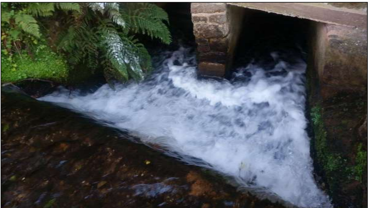
Figure 7: The weir immediately upstream of Town Mills
