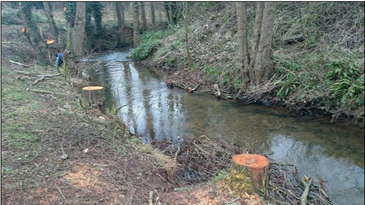
Figure 27: Small brushwood berms introduce flow diversity into a small stream
