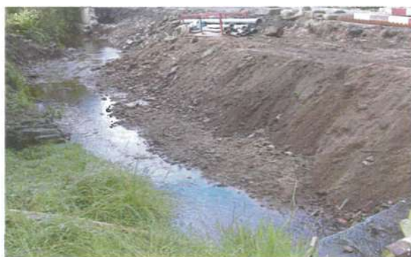
Channel after removal of wall - 7 th July 2000
