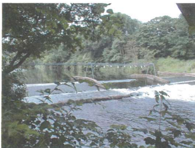
Fig 2 Corby Hill counter showing gantry with cameras over central channel
