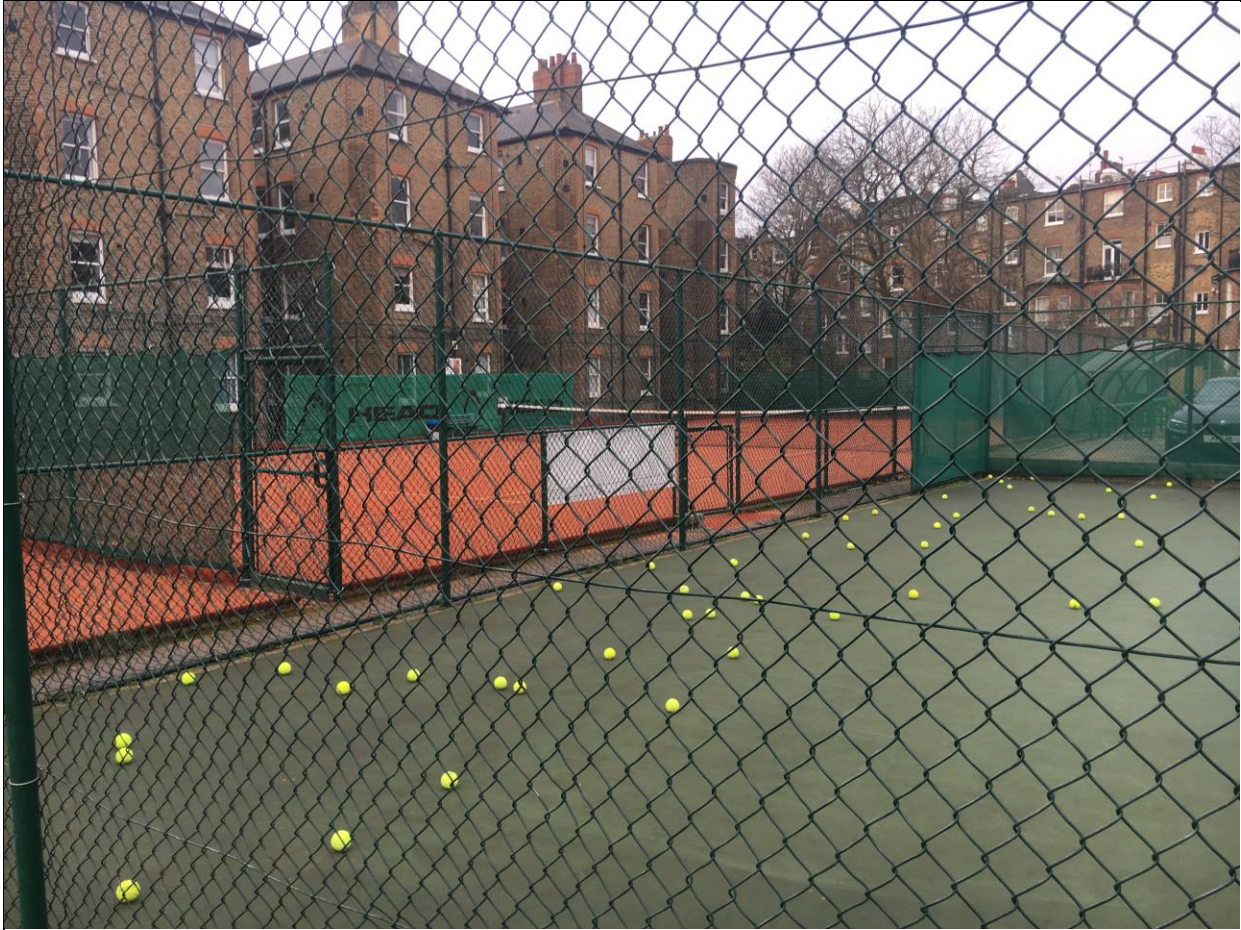
View looking to the rear elevation of Delaware Mansions
