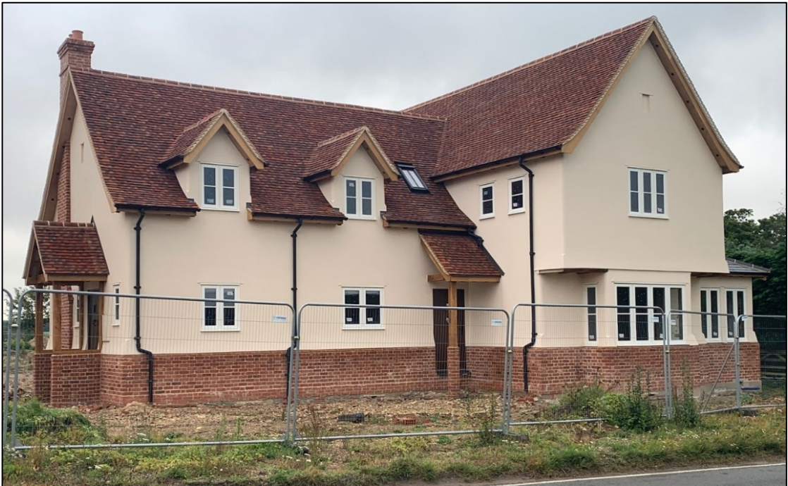
Figure 16: Homes under construction at Well Court in Hunsdonbury reflect roof lines and dormer features
