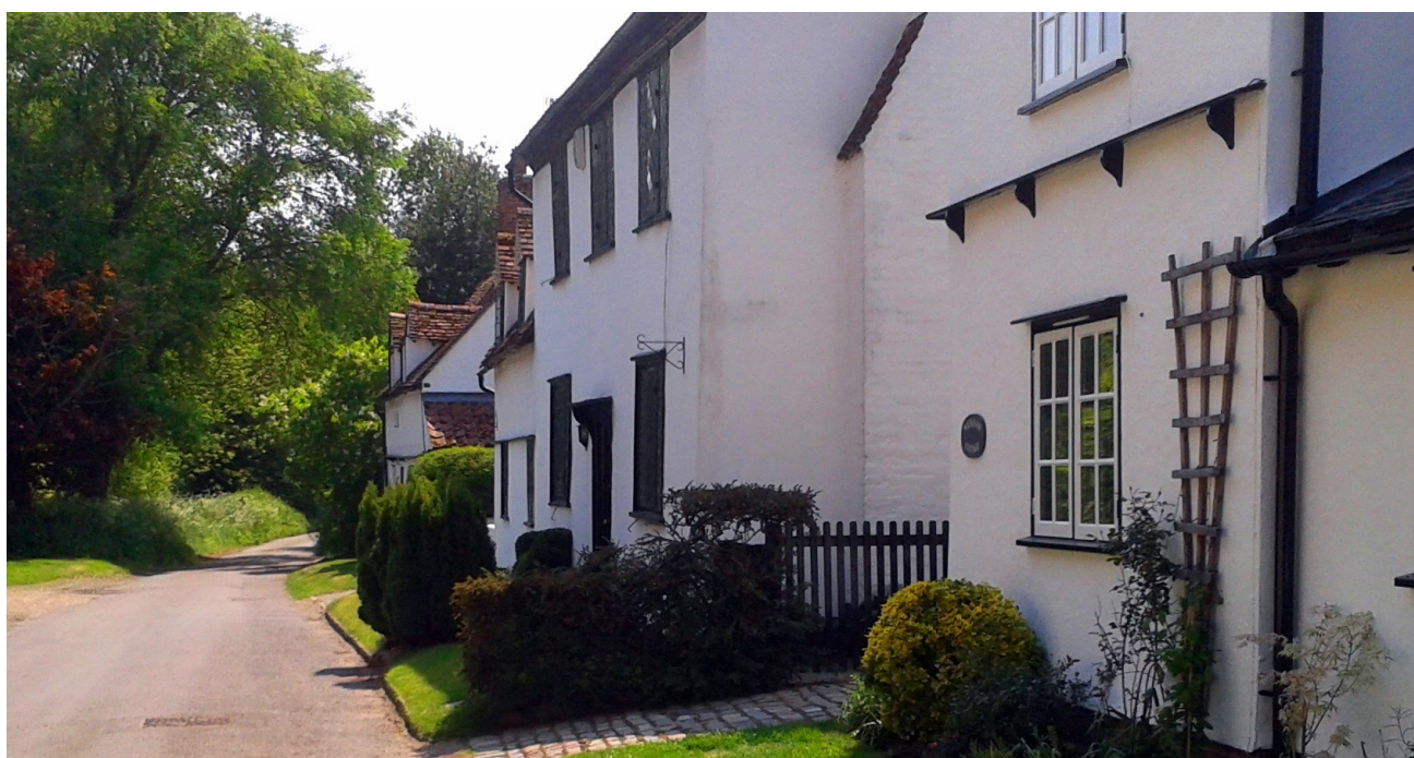
Figure 5 Grade II listed cottages, Church Lane
