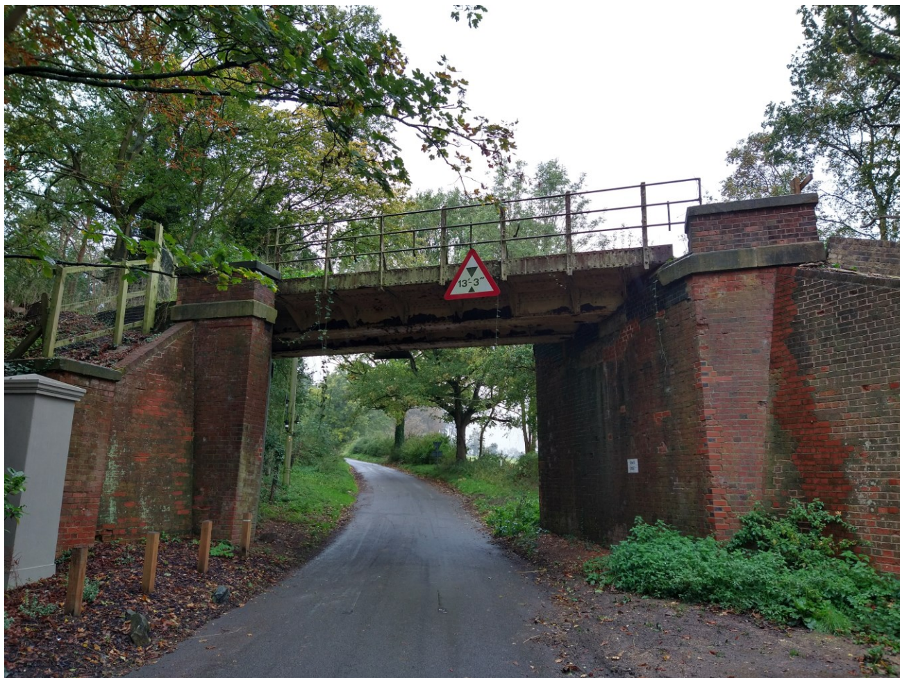
Figure 25 Blackbridge Lane Bridge
