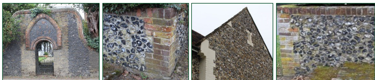
Figure 13 Examples of use of flint and brick in combination in Much Hadham
