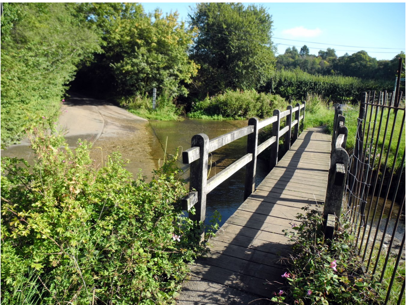
Figure 26 Footbridge over the River Ash
