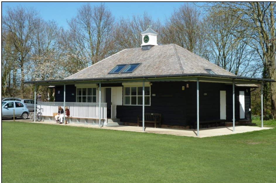
Figure 21 Sports Pavilion at the Recreation Ground
