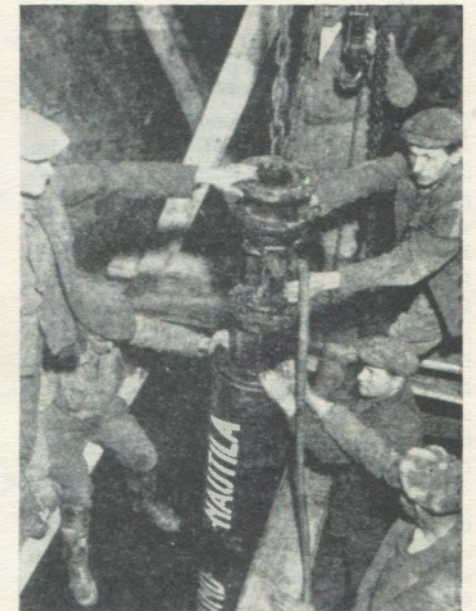
Figure 4. Installing one of the 'Nautilus' pumps in the Punkva Cave. Photo by Karel Absolon.
