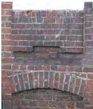
Parapet with a projecting gauged brick band, and flat window arches at Mull Cottage. The enlarged carriage entrance cuts through a blind window. ►
