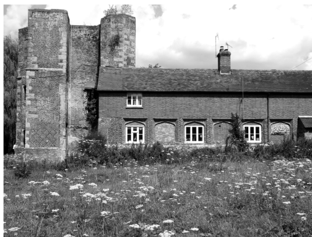
Fig. 12.7: The north-west tower and part of the surviving north range of Otford Palace, Kent. Photo by Matthew Johnson.
