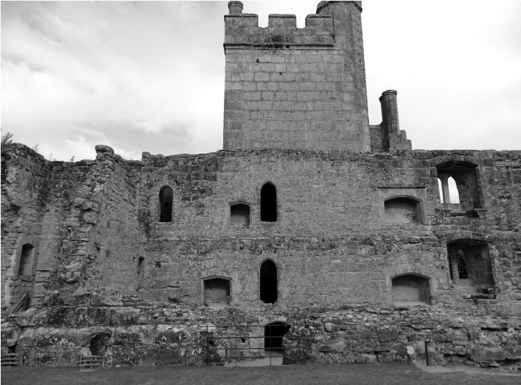
Fig. 9.2: The eastern elevation of Bodiam Castle, taken from the west. Photo by Penny Copeland.
