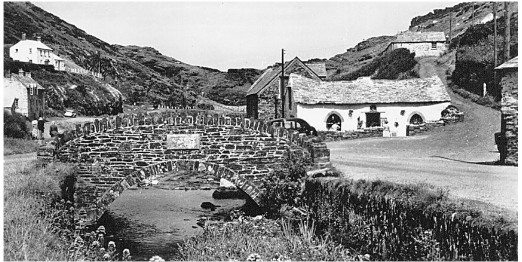
the Lower Bridge as it looked before being damaged by the 2004 flood
