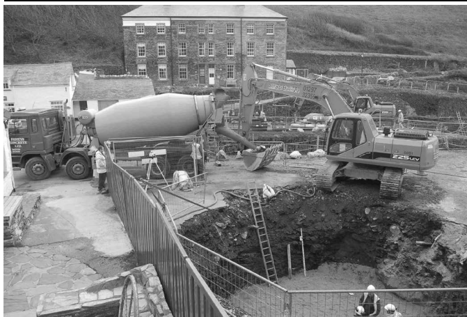
construction work continued around the village
