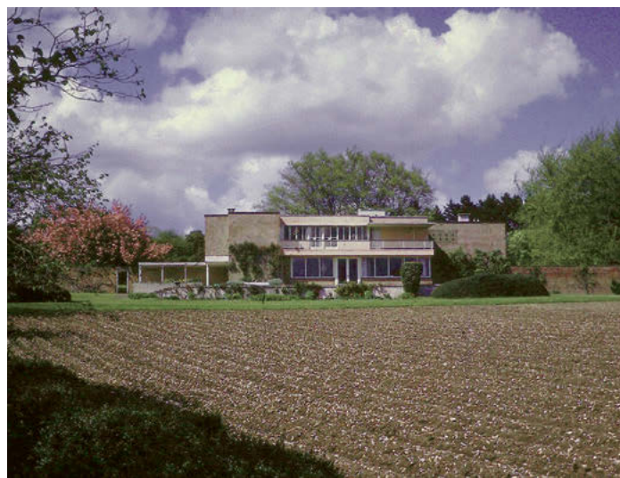
(Above) The Wills' home, a Kit Nicholson-designed house bearing a resemblance to the Dunstable clubhouse designed by the same architect
