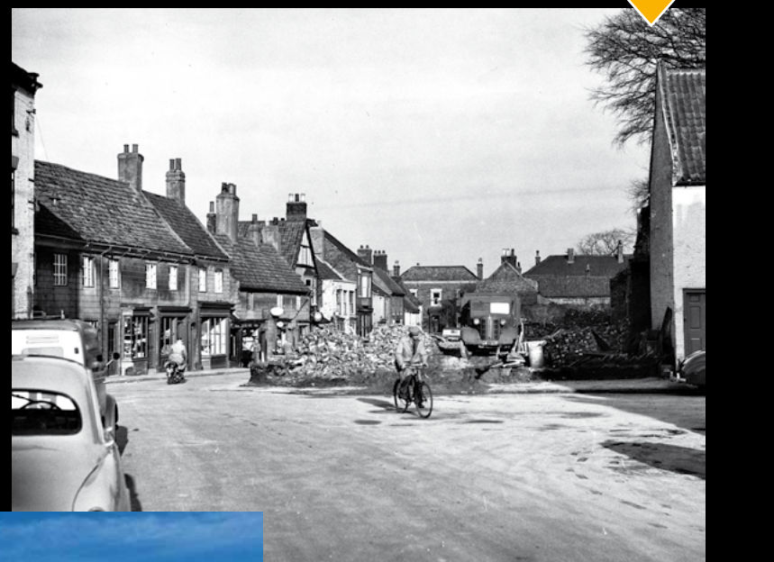
The demolition of Priestgate House in 1954
