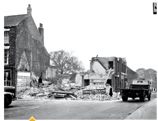
Buildings in Market Lane during demolition
