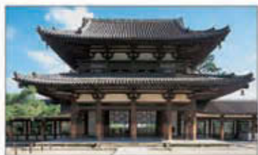
Gate at the Horyu-ji compound
