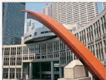
Tokyo Metropolitan Government Offices This huge complex of two blocks and a semi-circular plaza is unified by the grid-detailing on its façades (see p88), recalling both traditional architecture and electronic circuitry. An observatory gives views from Mount Fuji to Tokyo Bay on a clear day.
