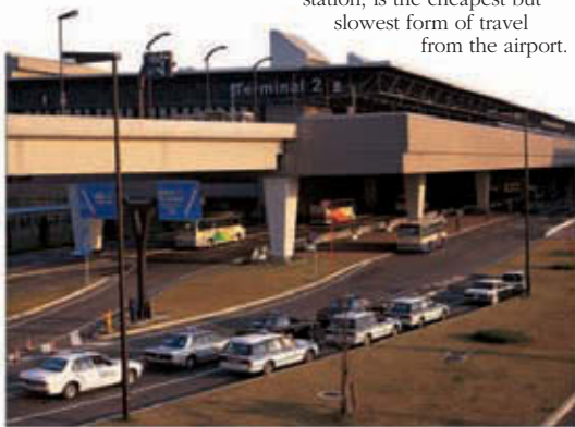
Terminal 2 of Tokyo New International Airport, at Narita
