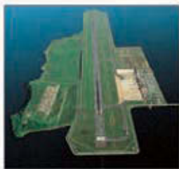
The runway of Nagasaki Airport, built on the sea
