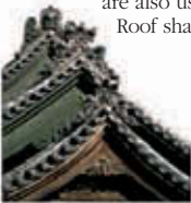
An intricate, gabled roof with decorated tile ends
