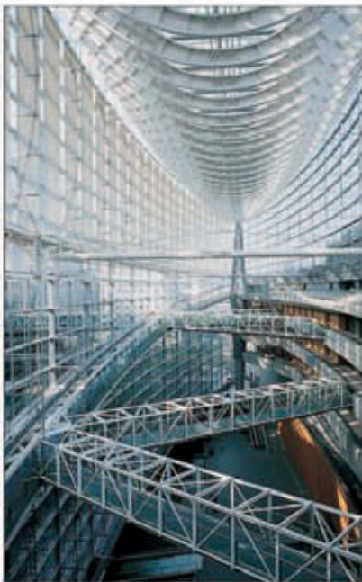
The airy glass-and-metal interior of the Tokyo International Forum
