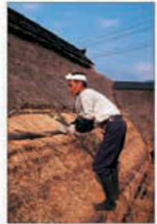
A thatcher at work replacing worn thatch
