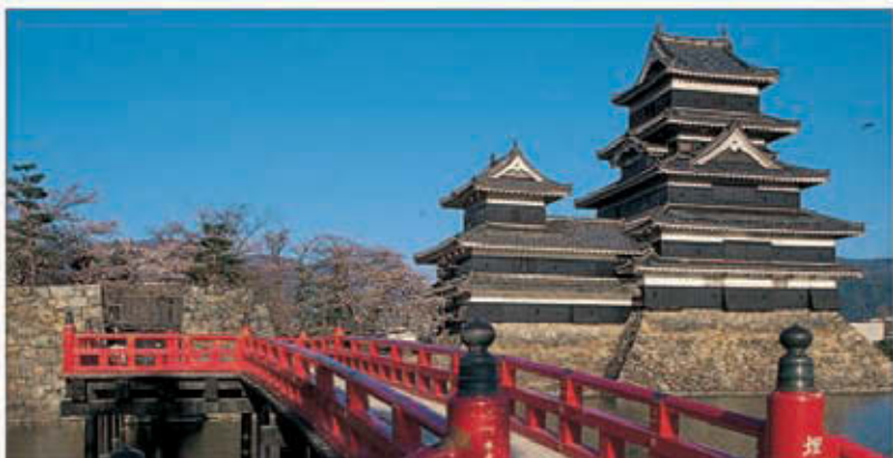
Bridge leading to the immaculately preserved Matsumoto castle
