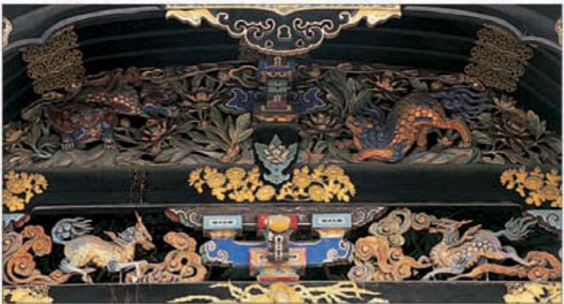
Detail of the main gate fronting the street at Nishi Hongan-ji
