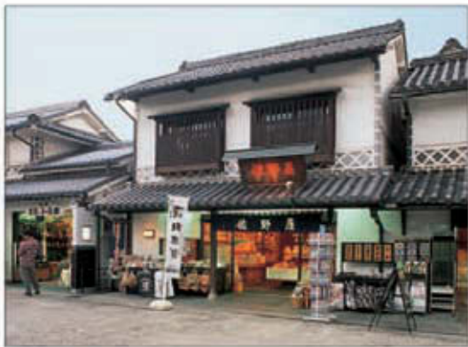
One of Kurashiki's storehouses, now a shop
