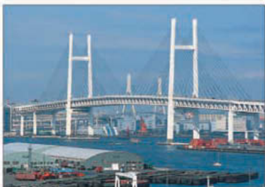
Yokohama Bay Bridge
