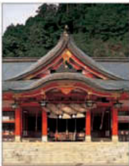
Taikodani Inari Shrine in the town of Tsuwano
