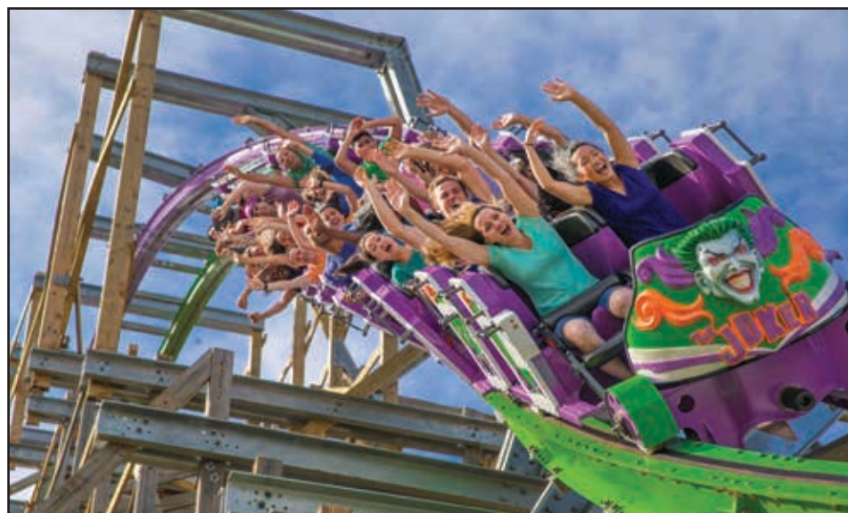
Like the DC Comics "Batman" villain for which it is named, the vivid green-and-purple track of The Joker — a steel-on-wood redo by Rocky Mountain Construction of the former coaster Roar — tears gleefully through the landscape at Six Flags Discovery Kingdom. COURTESY SIX FLAGS DISCOVERY KINGDOM
