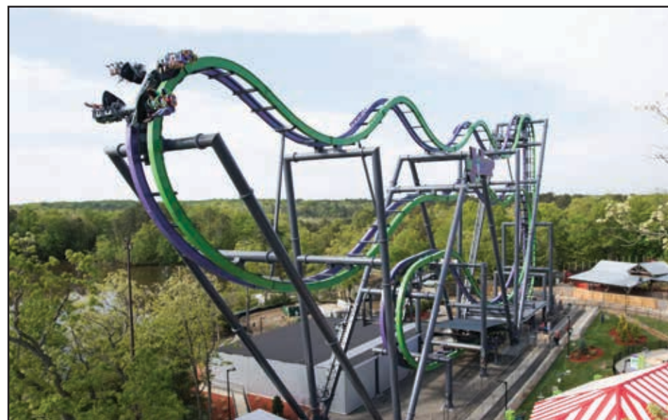
The Joker is Six Flags Great Adventure's newest roller coaster thriller. Sipped by Utah-based S&S Worldwide, the 4D Free Fly coaster never gives two identical rides, thanks to the individual spinning action on the vehicle's seats. COURTESY SIX FLAGS GREAT ADVENTURE
