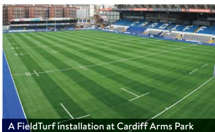
A FieldTurf installation at Cardiff Arms Park
