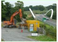
National Rail- Now you may wonder what the "new road" is for, in the field alongside the High Path? Apparently there are some drainage issues north of the railway station. New drains need to be laid and the road, made of 4000 tons of recycled hard-core, is to facilitate access to the site for the heavy plant needed to do the work. This is expected to take 10 -12 weeks.
