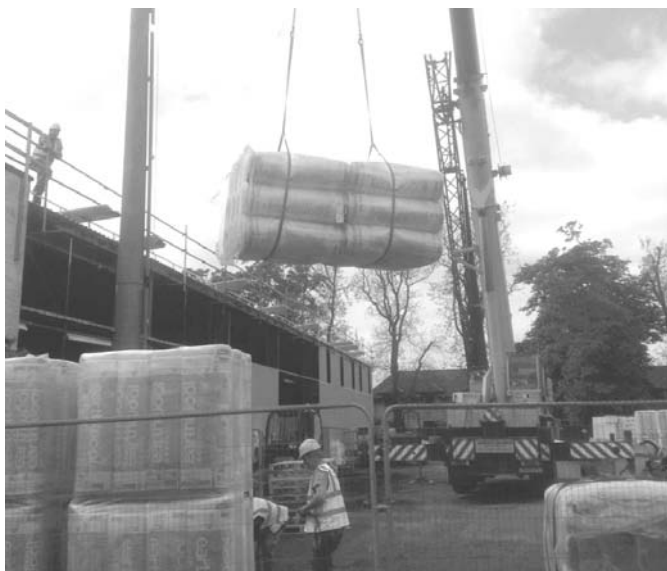
Rolls of insulation for the roof being delivered photo: Donald MacGregor
