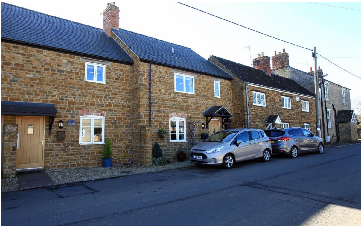
Infill development in Earls Lane, Deddington
