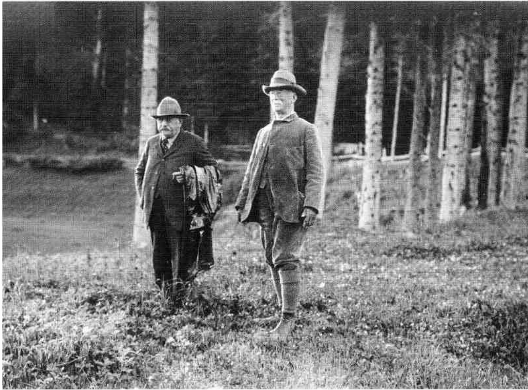
Archibald Mitchell (right) and his son-in-law Edward Alan Olds (left) surveying the site for the "New Camp" (Runnymede Lodge).
