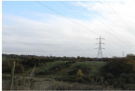
View of southern slope of dry valley with power line on plateau
