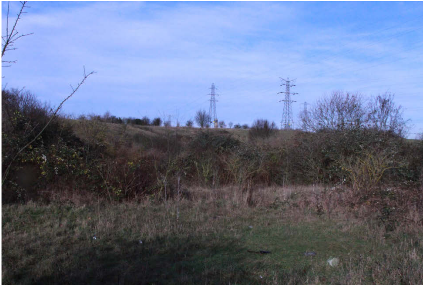
Northern slopes of the dry valley, with low voltage power lines on plateau
