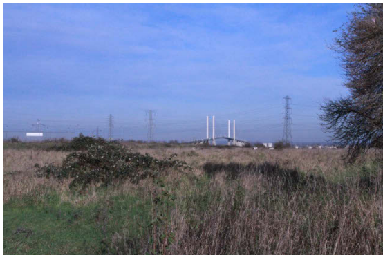
View of QEII Bridge from Area 1
