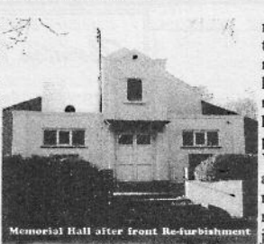
Memorial Hall after front Re-furbishment
