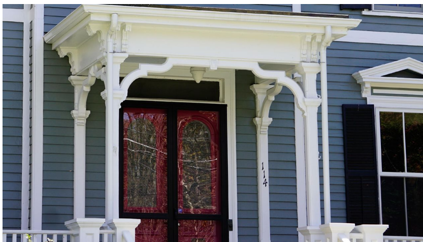
Example of Italianate style: Entry of the Gardiner Gates House (1874) at 114 Temple Street
