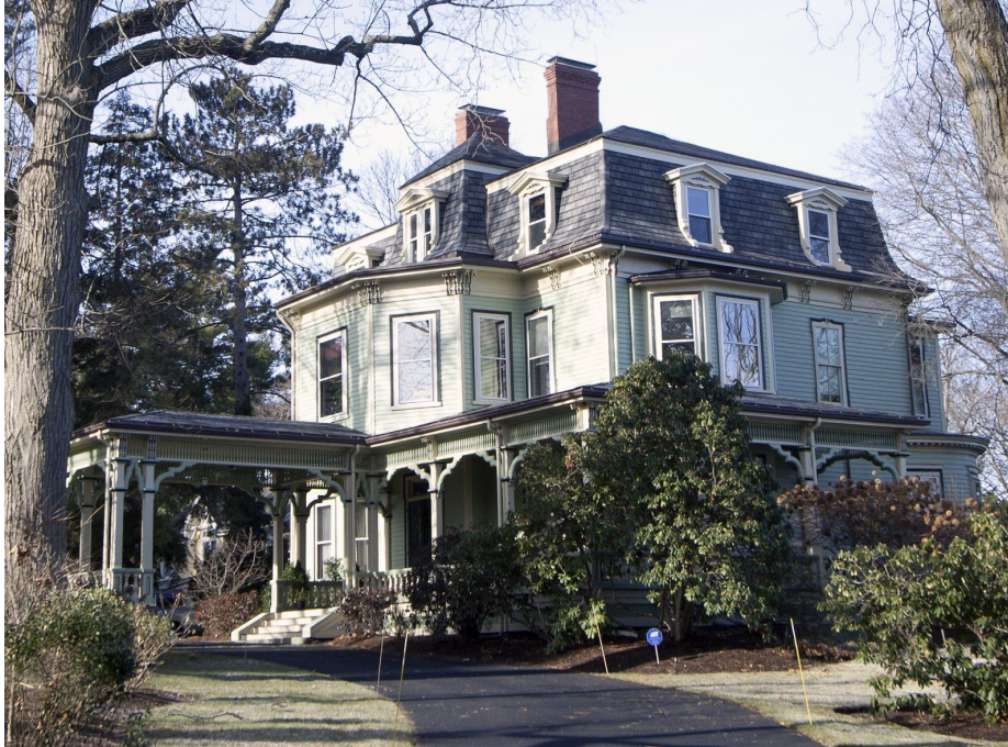
Example of Second Empire Style: David Howland House (1873) at 129 Chestnut Street
