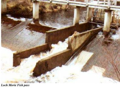
The weirs at Loch Morie and Dalmore Distillery are both provided with fish passes which appear to be effective for both upstream and downstream passage. A poorly designed fish pass and culvert on a main tributary at Boath should be dealt with under CAR regulation.
