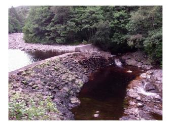
Just above Orrin Falls there is a weir and lade which supplies a private hydro scheme at Fairburn House. The weir is made passable by a diagonal dished channel fish pass.
