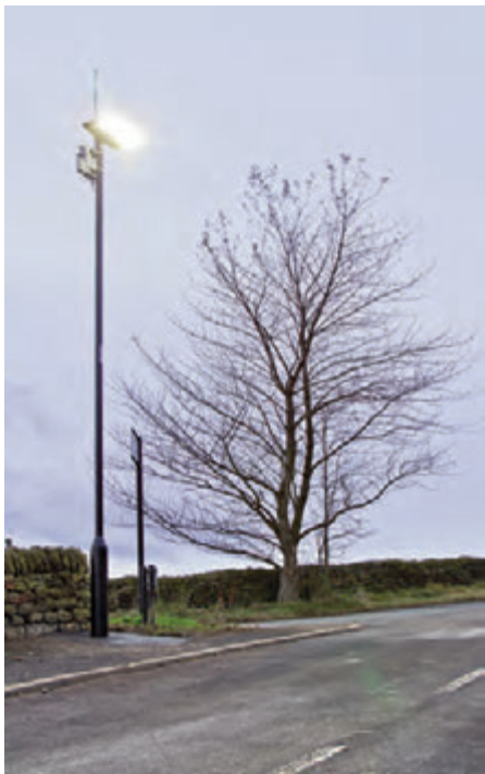
The new LED lights direct light down onto the road surfaces and so reduce light pollution.
